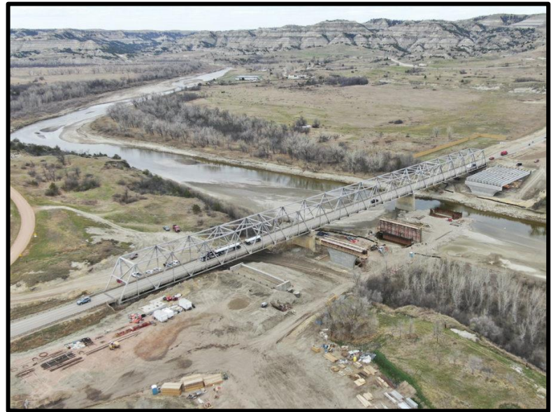
Figure 4-26: Long X Bridge and New Replacement Bridge
