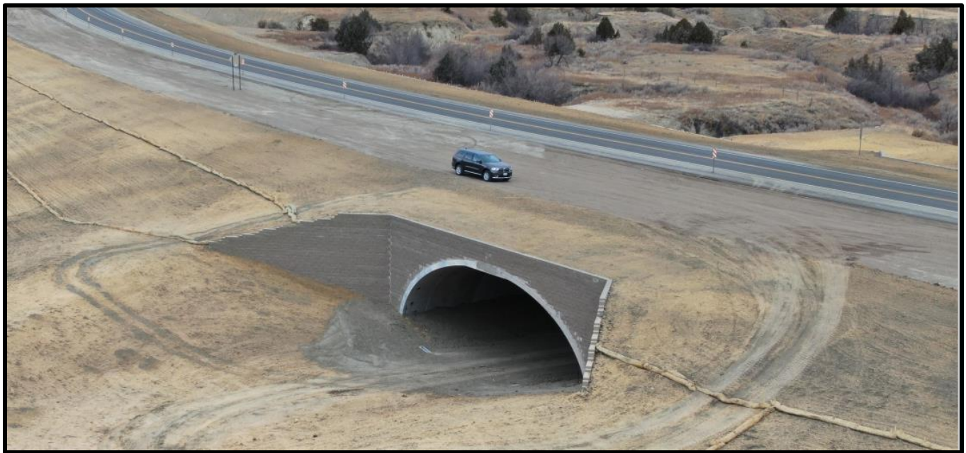
Figure 5-25: US-85 Wildlife Crossing
