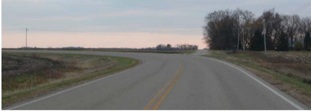
FIGURE 2-9 Example of a Visual Trap – Minor Road Intersects Roadway on a Curve
