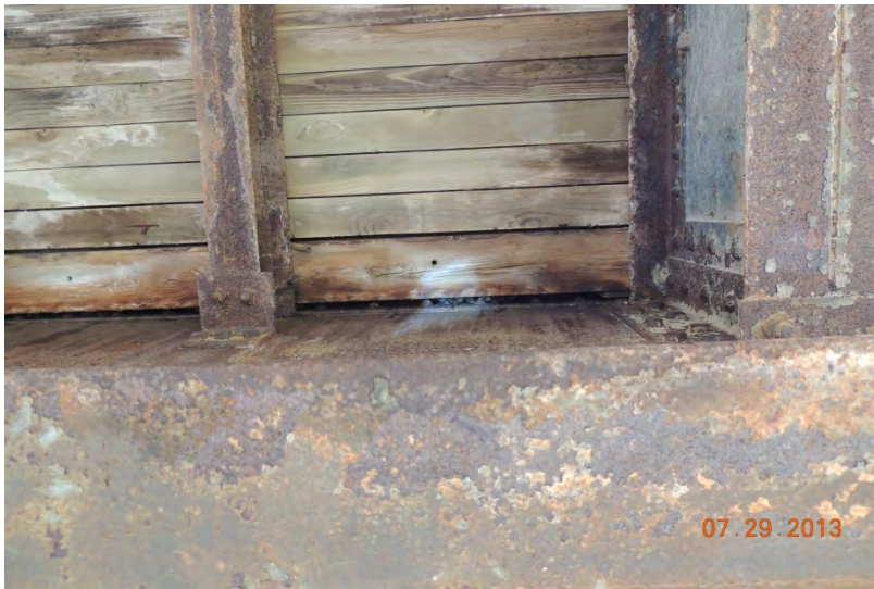
Photo 14: NLEBs roosting under a timber decked bridge
