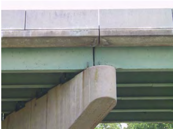
Photo 3: Example of open concrete joint used by bats
