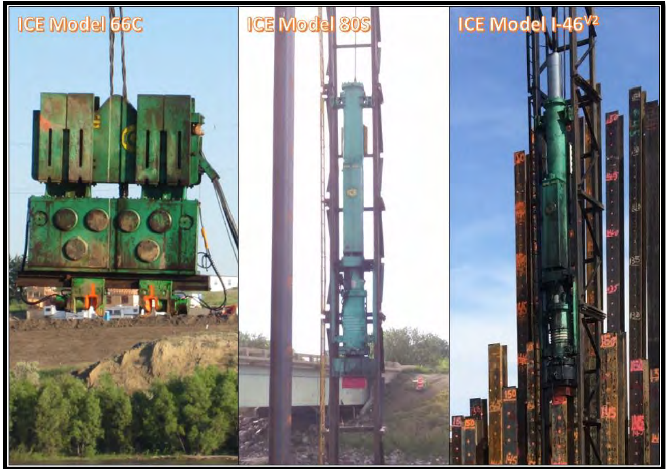
Figure 3, Vibratory and Impact Hammers
