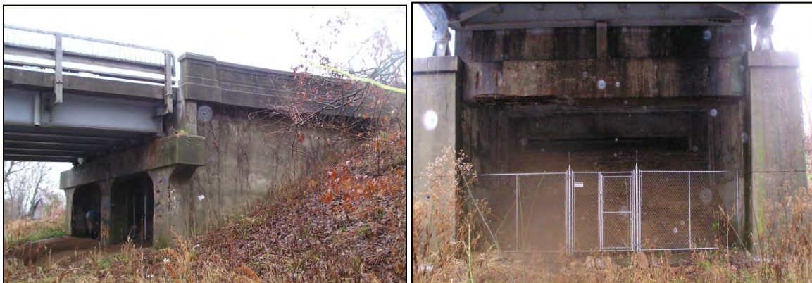
Photo 12 and 13: Bridge design mimicking “cave-like” atmosphere
